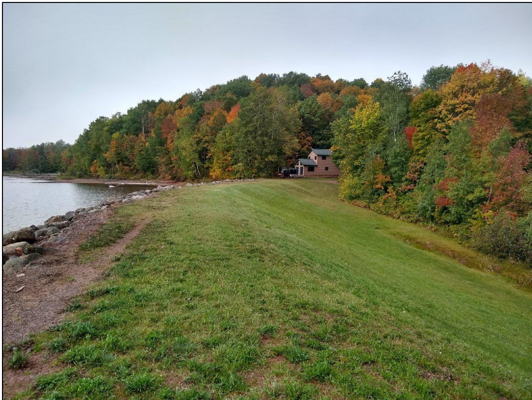
Figure 3.10.1-2 View of Gile Dam Looking West
